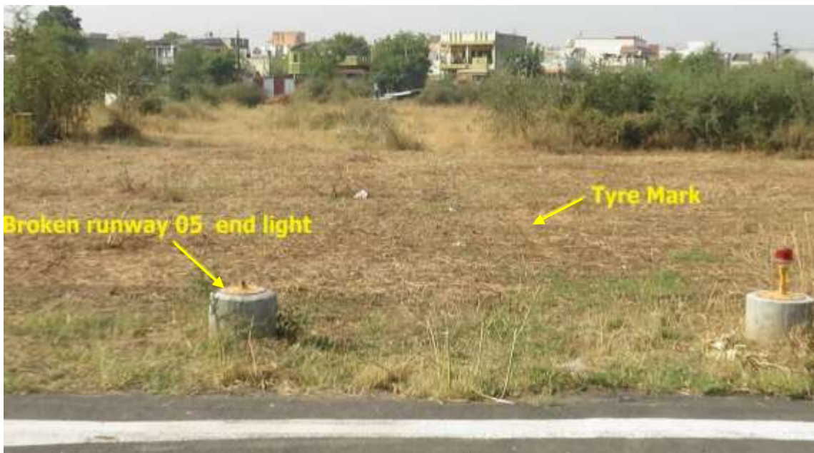
Image 28. LH wheel of aircraft ran over runway end light
