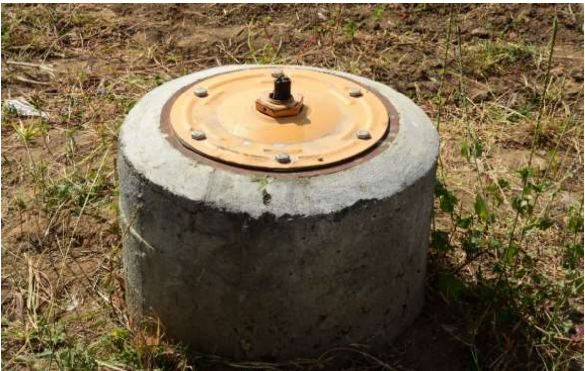
Image 20. Broken runway end light
