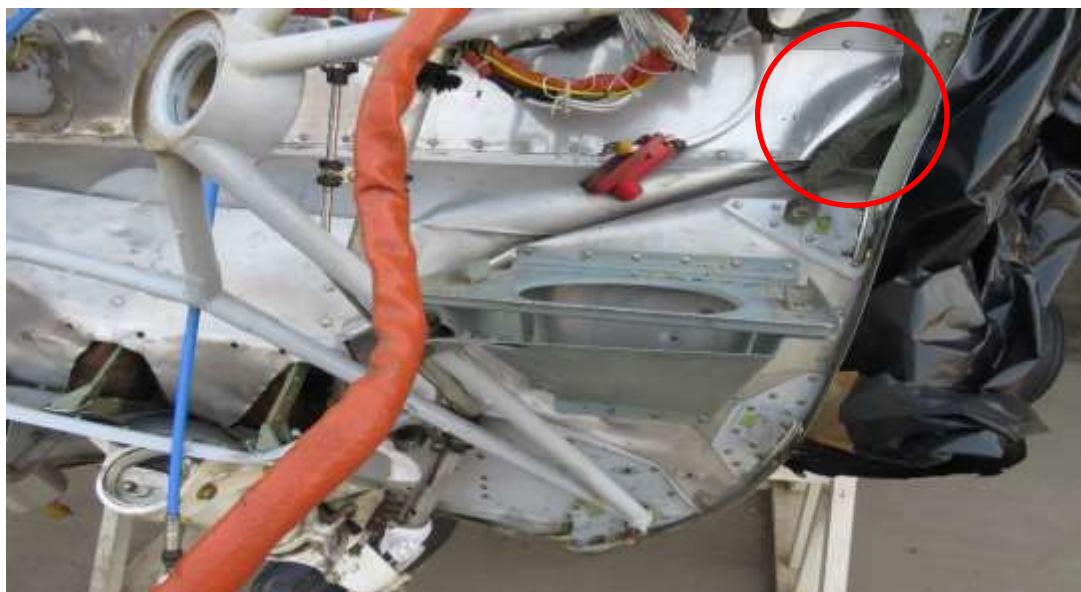
Image 18. Damage to upper firewall
