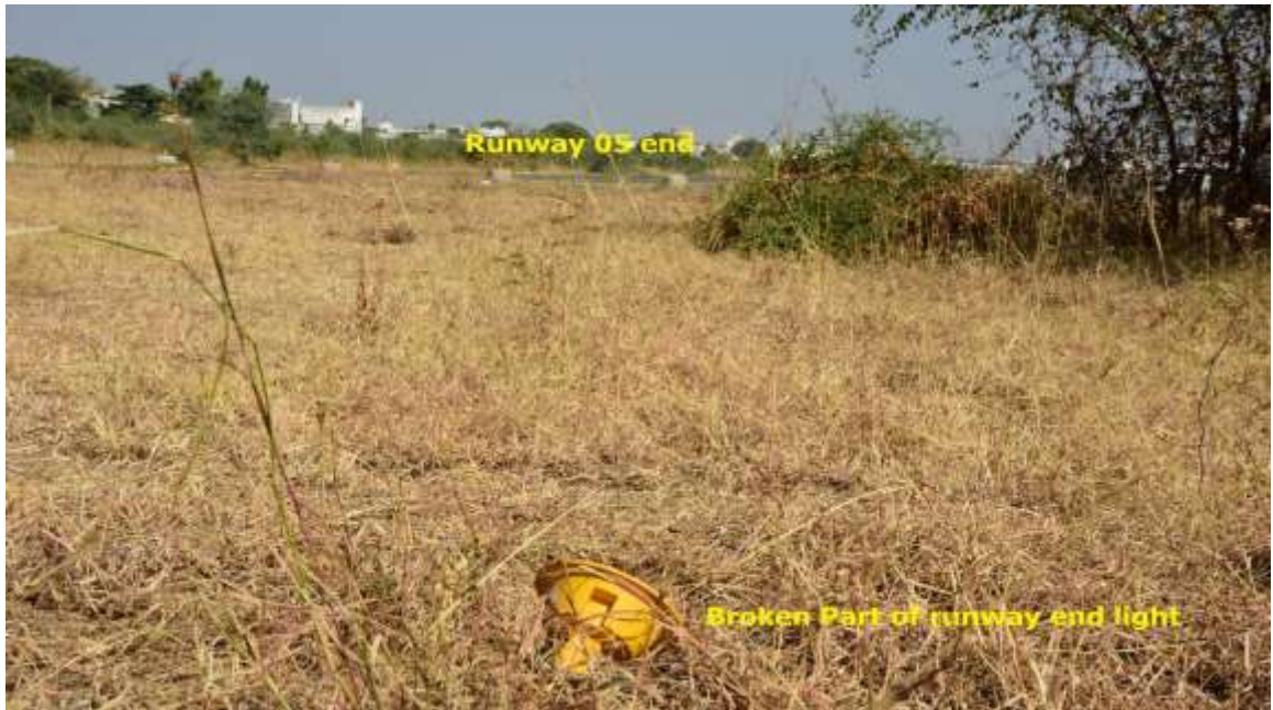
Image 29. Broken part of runway end light found on unpaved surface
